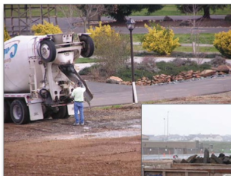
Figure 1. Chute washwater being dumped on the ground
