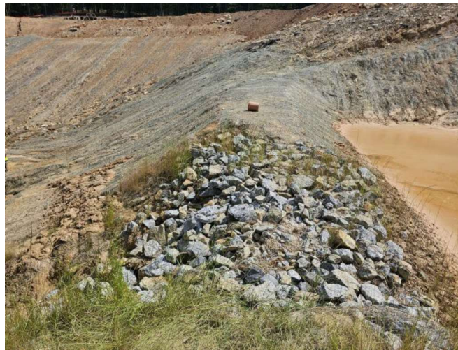
Rock dam at SD4C-8
