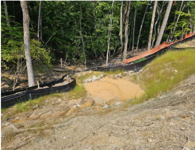
Sediment Basin SD3-7 looking down stream
