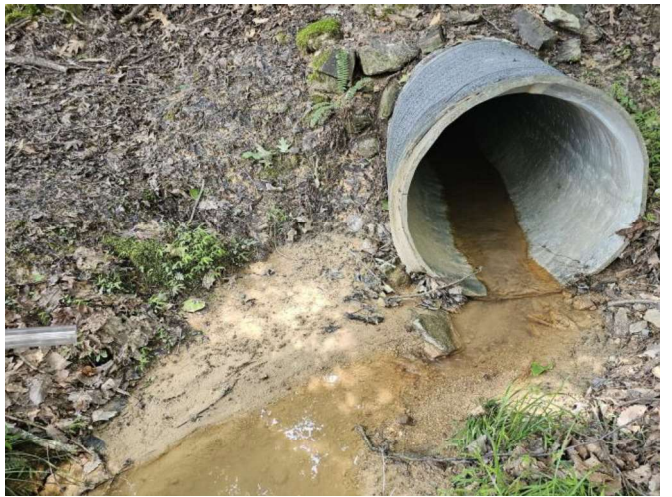
Downstream of Station A-11
