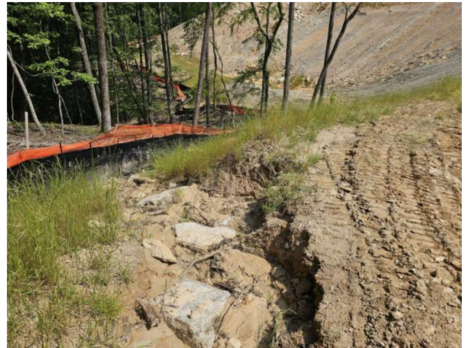
SD1-S looking southeast towards SD3-7
