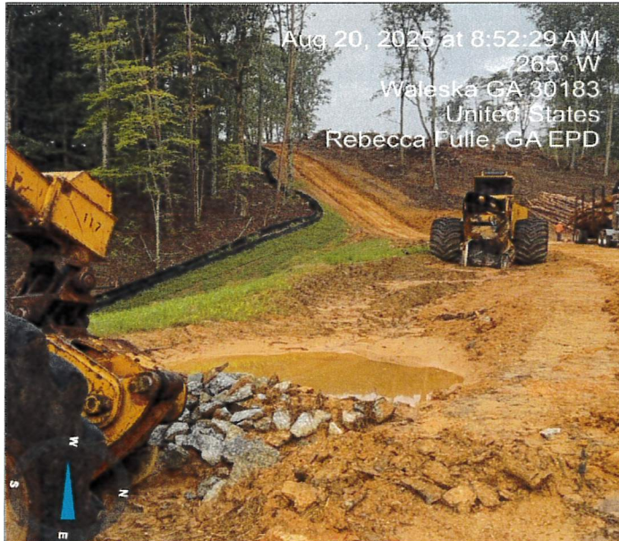
Photo Number: 1 of 6 Date: 08-20-25 Photographer: Rebecca Fulle Location: Site, facing West Observations: Heavy machinery parked on top of a diversion.
